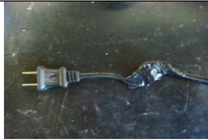
Cover the entire thing in electrical tape or shrink tubing.
